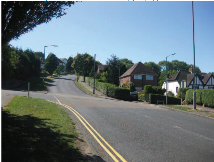
Photo 3.1: Braybon Avenue, southbound (uphill) approach to crossroads
